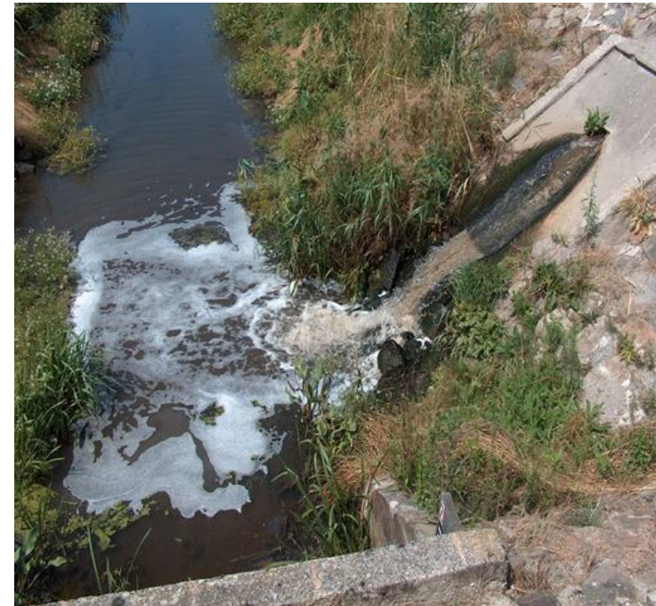
Waste Water Treatment Plant
