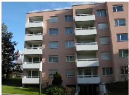
Building facade (painted with the same product as the new facade)
